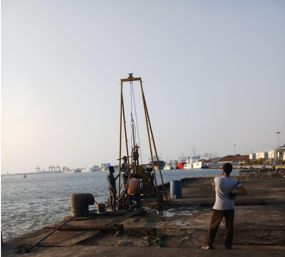
Figure 25 A view of Geo Technical Investigation at South Coal Berth
