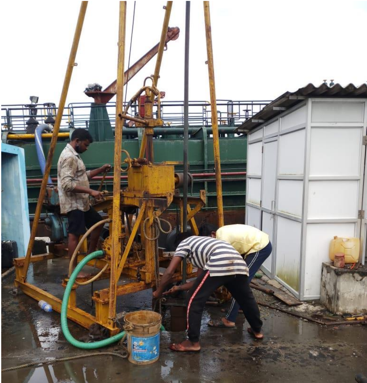
Figure 24 A view of Geo Technical Investigation at South Coal Berth
