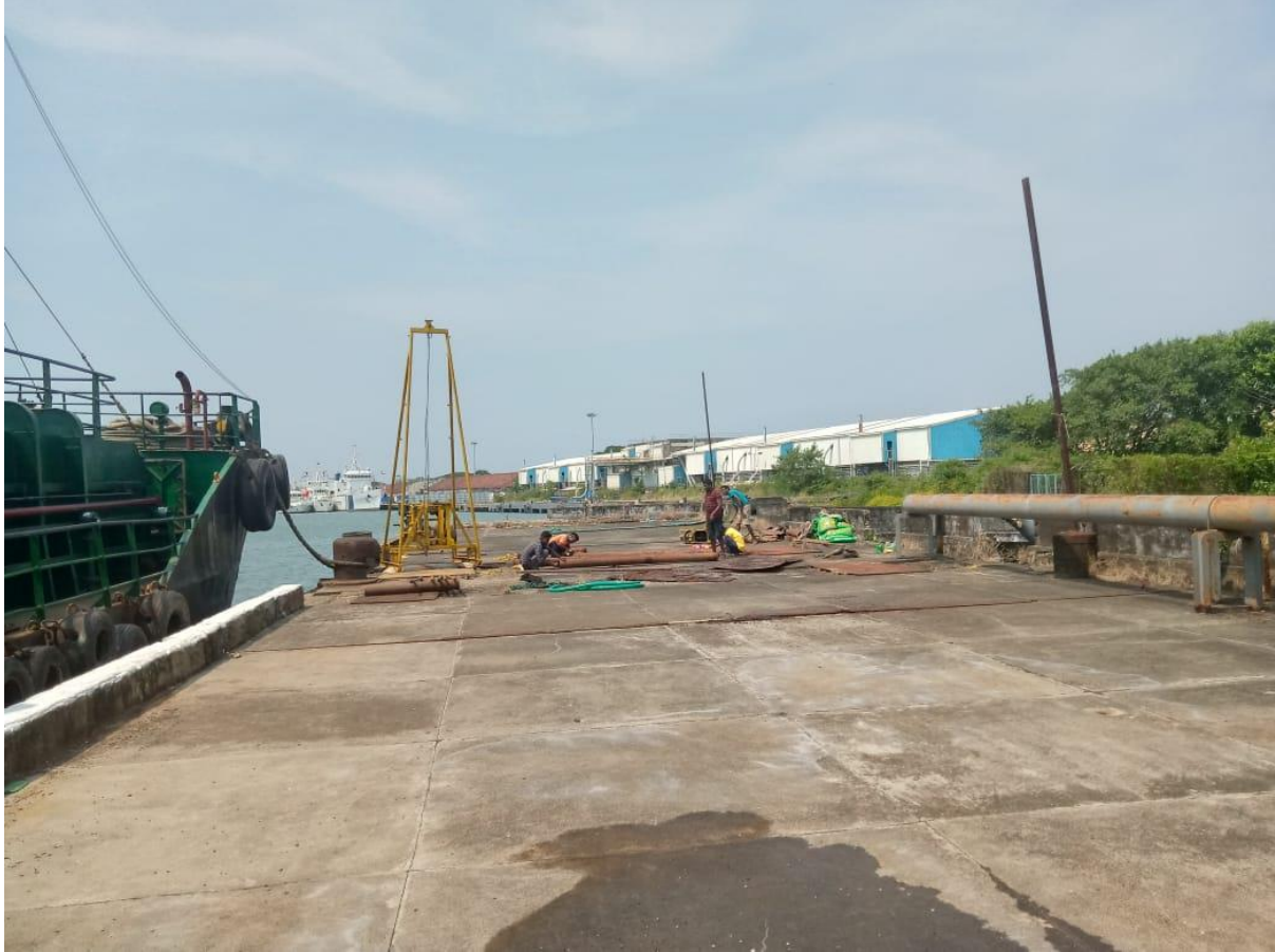
Figure 23 A view of Geo Technical Investigation at South Coal Berth
