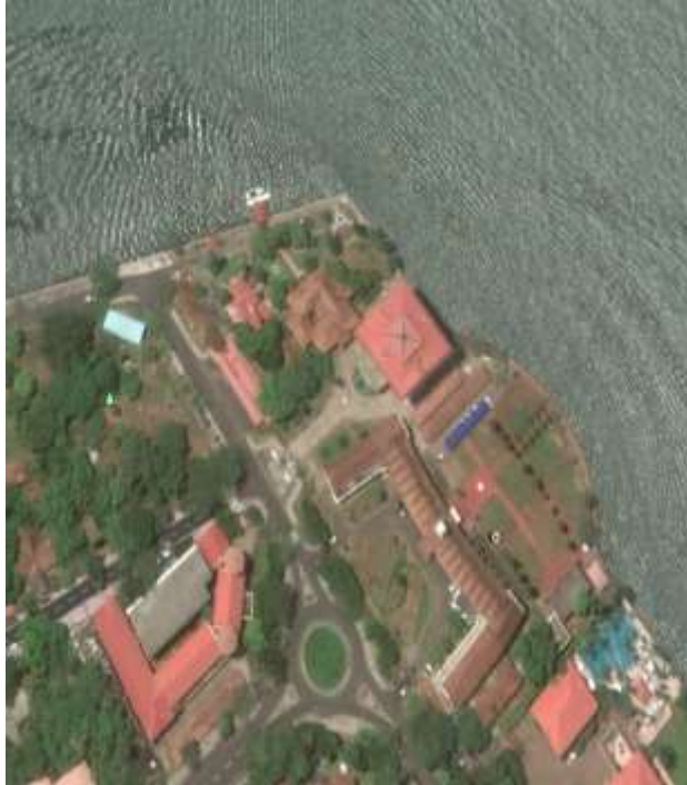
CPT (Admin Office)
